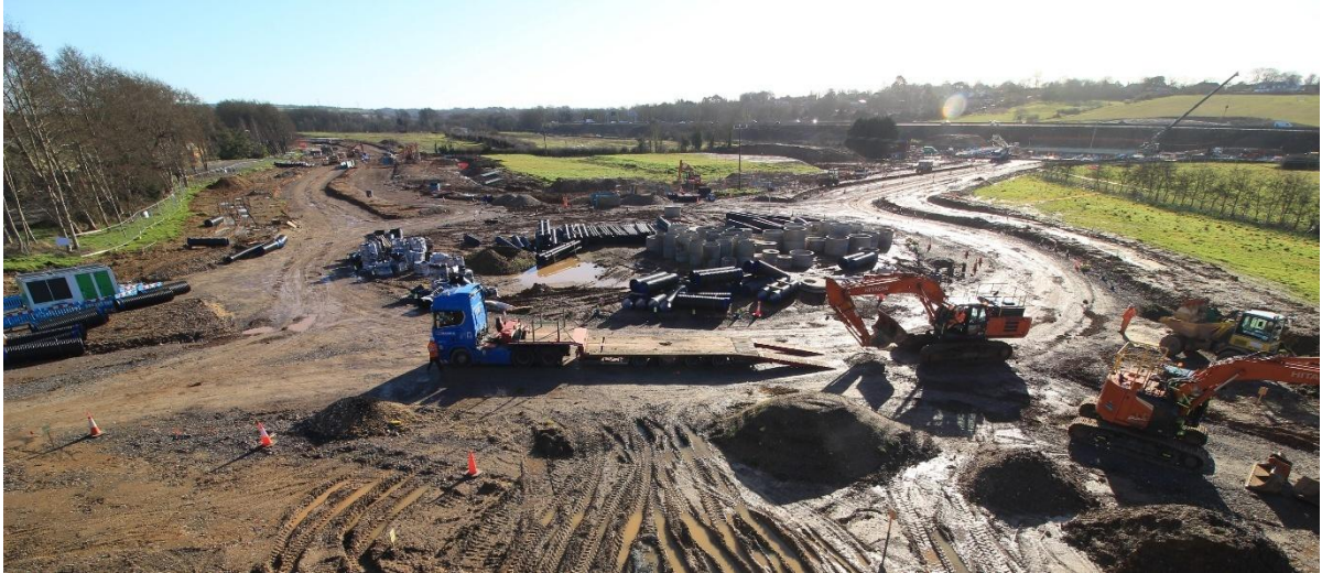
Construction of the Welborne Approach Roundabout
